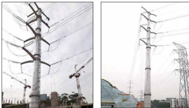
Monopole pylon towers
